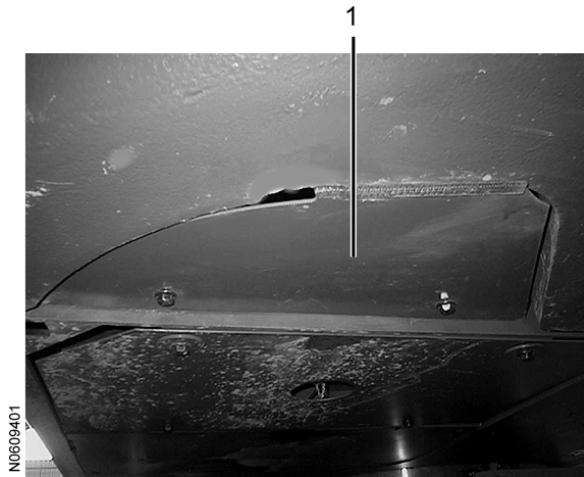
Figure 3 Inspection cover, underside of counterweight
